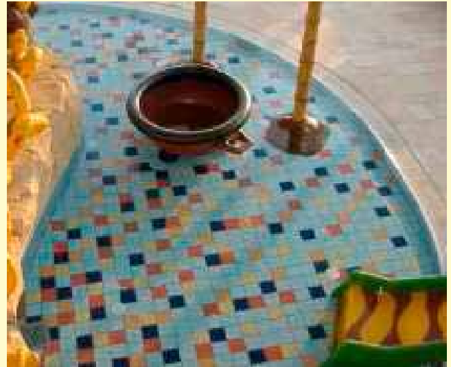
Children's splash pool with colourful design in the required slip resistance C
